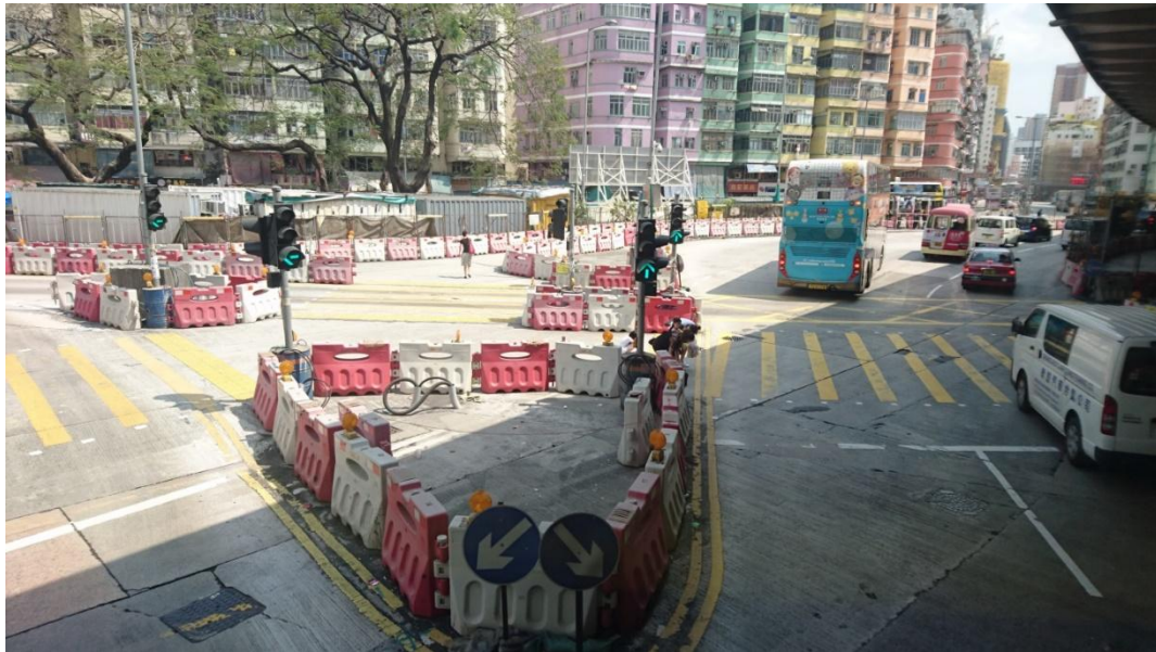
Figure 3.5.9: Temporary traffic management scheme in To Kwa Wan (Photo taken by Tang)
