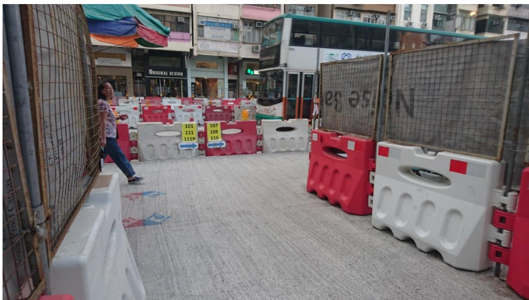
Figure 3.5.8: Relocation of bus stops on Ma Tau Wai Road (Photo taken by Tang)
