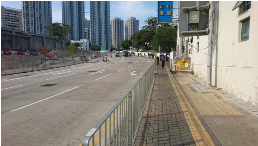
Figure 3.4.4: Nam Long Shan Road outside Wong Chuk Hang Station (photo taken by Tang)
